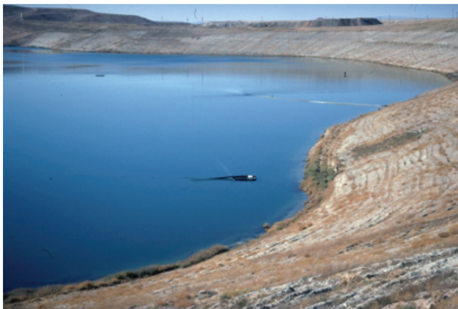
Figure 7 Re-graded final pit slopes at the Sleeper mine.
